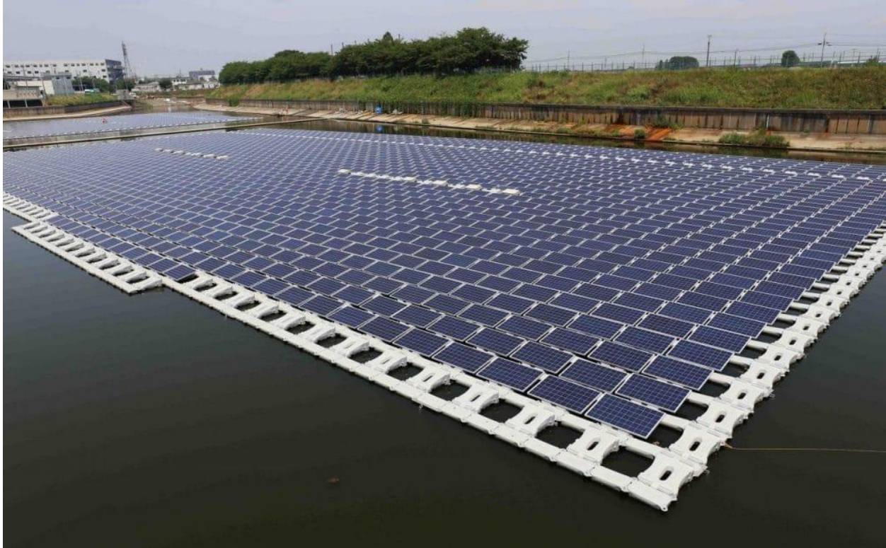
Fig. 1. A Floating solar PV plant. Source: Simemis. This figure shows the design of a traditional floating solar PV plant. This consists of many solar panels which are floating together connected within a floating base. All of them work together to produce combined power output.
